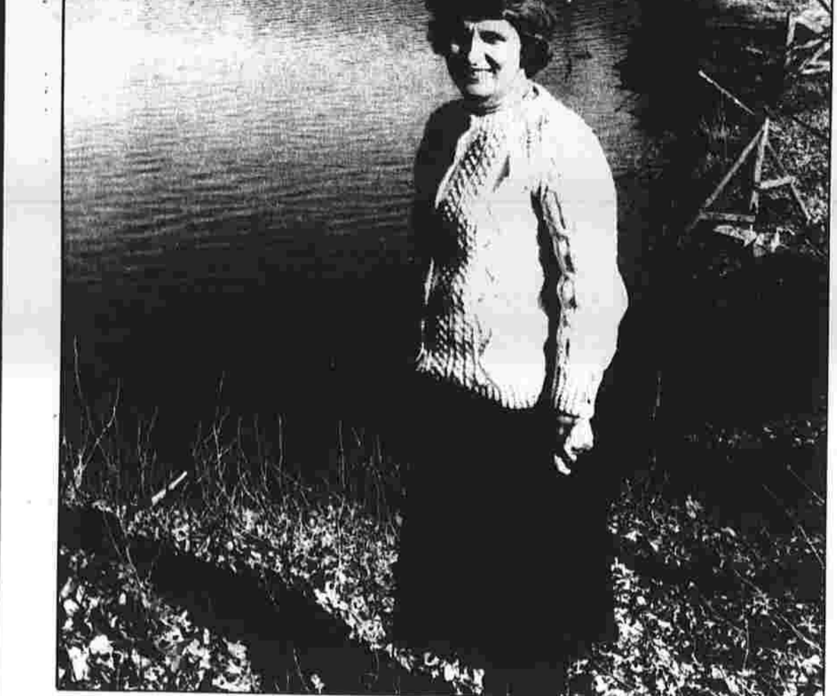
DAM DEMISE — Terry Parla, president of the Manchester Land Conservation Trust, stands near the dam at Rialley Reservoir at the John Risley Memorial Park. The dam needs repair and the trust is seeking contributions to augment a $200,000 grant from the state's Department of Environmental Protection to pay for the repair. Contributions should be made to the MLCT at 20 Hartford Road, Manchester 06040.
